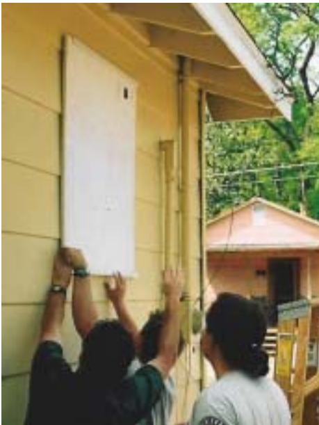
Shuttering is the most effective way to keep flying debris out.
