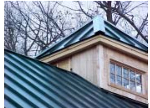
Standing-seam metal roofs do well when properly installed.
